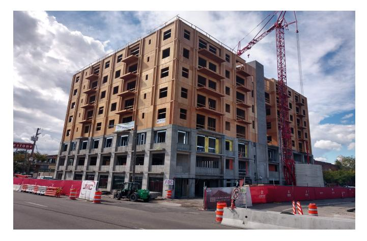
Figure 2. Structures like this 5-over-3 podium building near Salt Lake City, Utah, can use wood harvested from the WUI to provide dwelling units in increasingly densified urban corridors while helping to reduce standing tree densities in nearby forests. This FRTW could also be used in structures built in the WUI, too.
